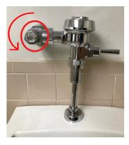
1.) Twist to remove the outer 2.) Turn the screw to either cover
