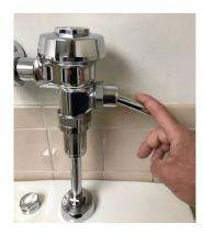
3) Flush to confirm the water flow has returned to normal
